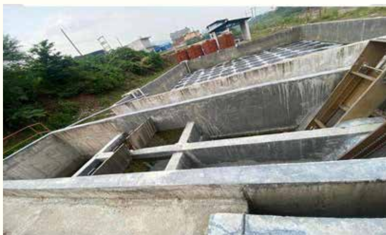
2C- Bar Screen Chamber 3C- Grit Chamber Mechanical
