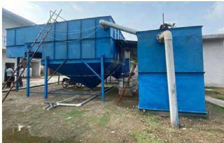
9E- PH- Neutralization Tank
